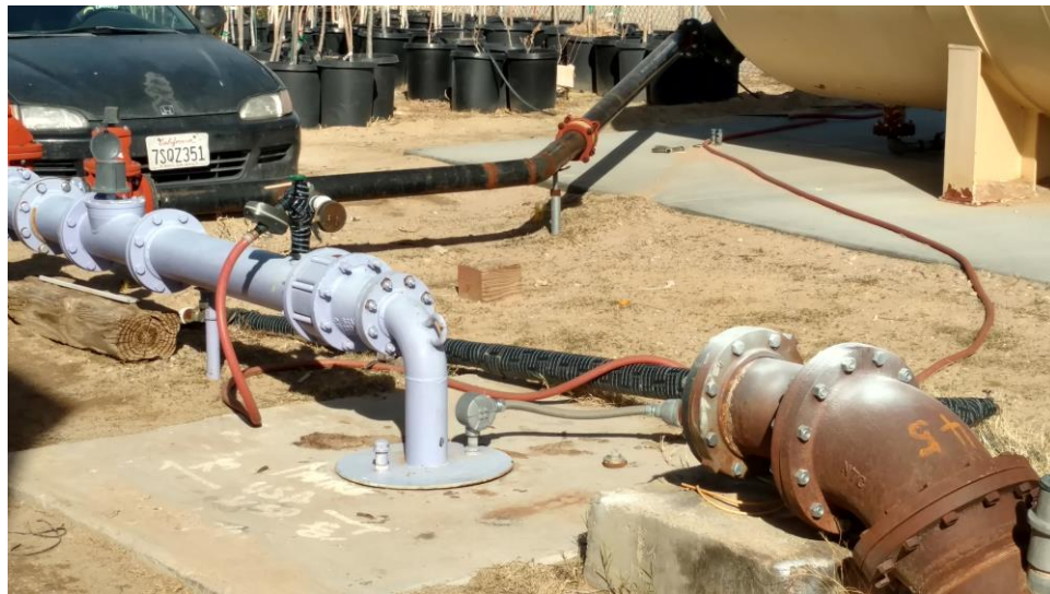
Maintenance Yard Area looking at Purple Pipe (Recycled Water)
