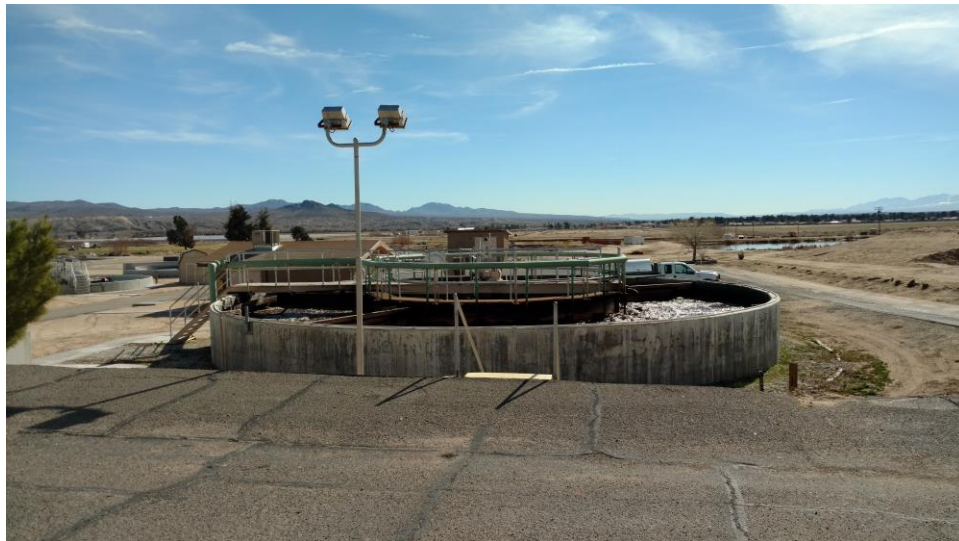
Helendale Community Services District – Wastewater Treatment Plant
