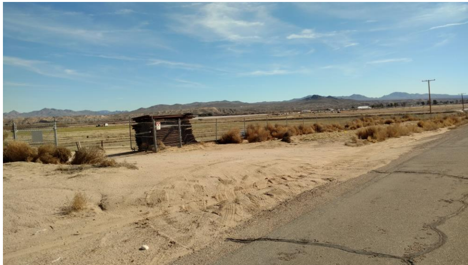
Helendale Community Services District – Wastewater Treatment Plant Field Area
