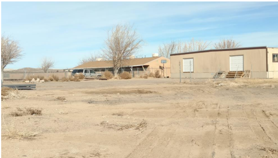
Maintenance Yard Area looking at 4-Plex and Potable Buildings
