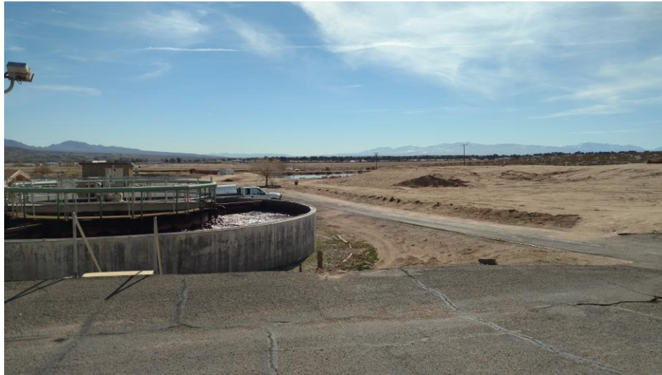
Helendale Community Services District – Wastewater Treatment Plant
